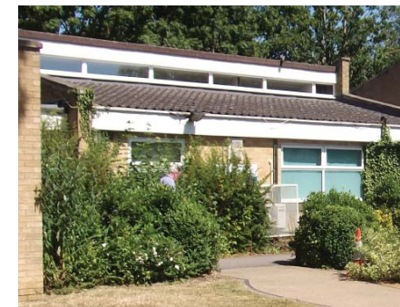
Figure 2.16 Health centre, Exeter Close
